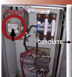
Safety is a big concern in all motor control centers. This Type W unit had a broken handle which was unsafe for personnel. A retrofitted unit is ready to install with all the safety features intact.
