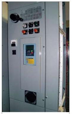
Variable frequency drives and can be installed <u>within</u> a motor control center as this Westinghouse Type W sample shows. A waste water treatment plant in Arizona had limited space and required a custom engineered solution utilizing a 'bubble' door.
