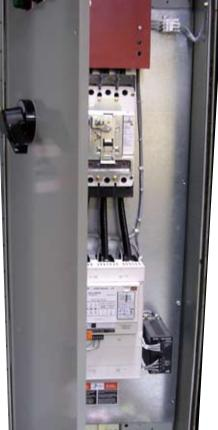
This soft-start retrofit for a 250 HP motor offers long term cost savings and reduced a tripping nuisance. Utilizing a custom backpanel approach the design reduced installation costs and minimized downtime, compared to a new MCC, and improved reliability.
